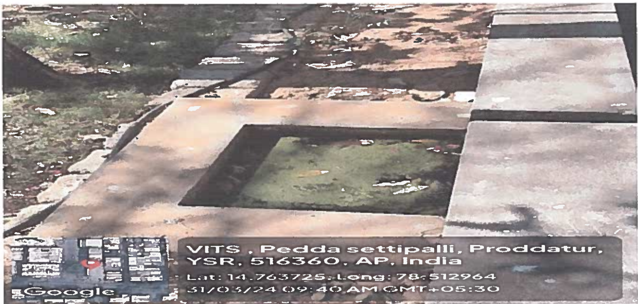
Rain Water Harvesting Pit – 1
