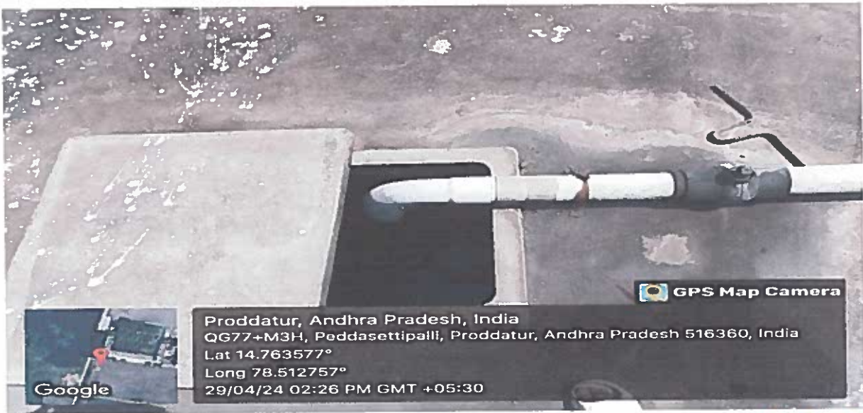
Water Recharge Pits at various Locations
